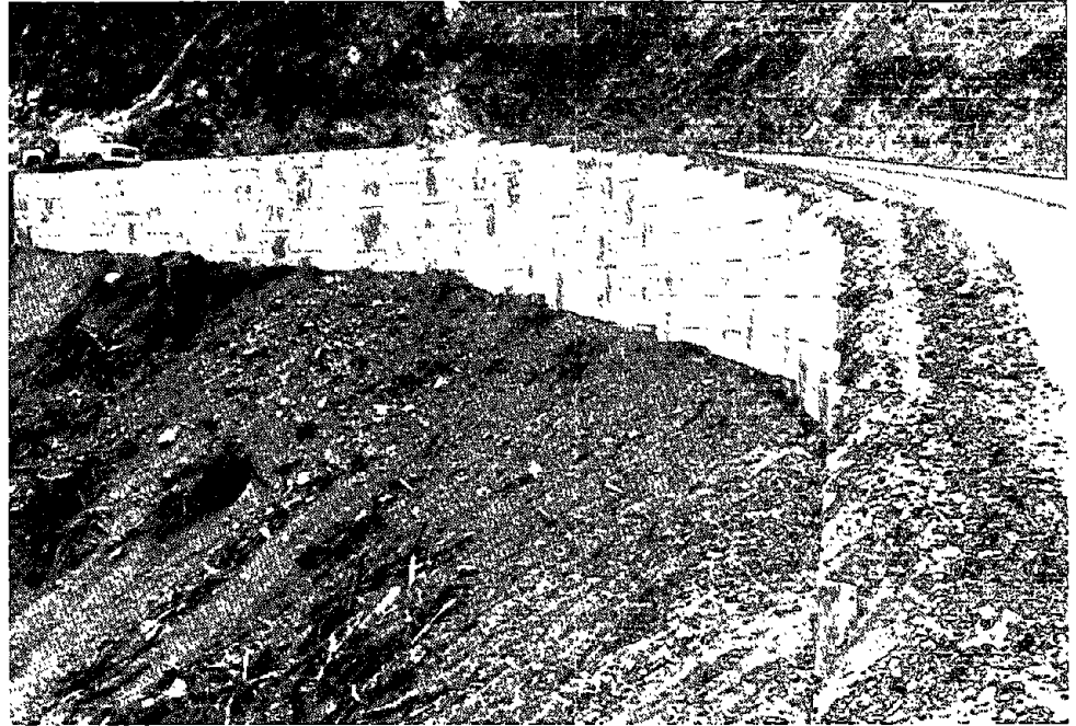
Figure 2-2.—Reinforced earth wall.
