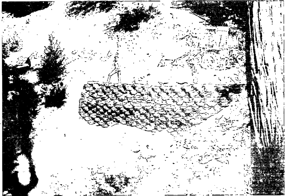
Figure 2-5.—Tire-Faced Geotextile Wall.
