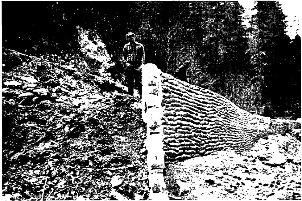
Figure 2-6.—Stack Sack wall.
