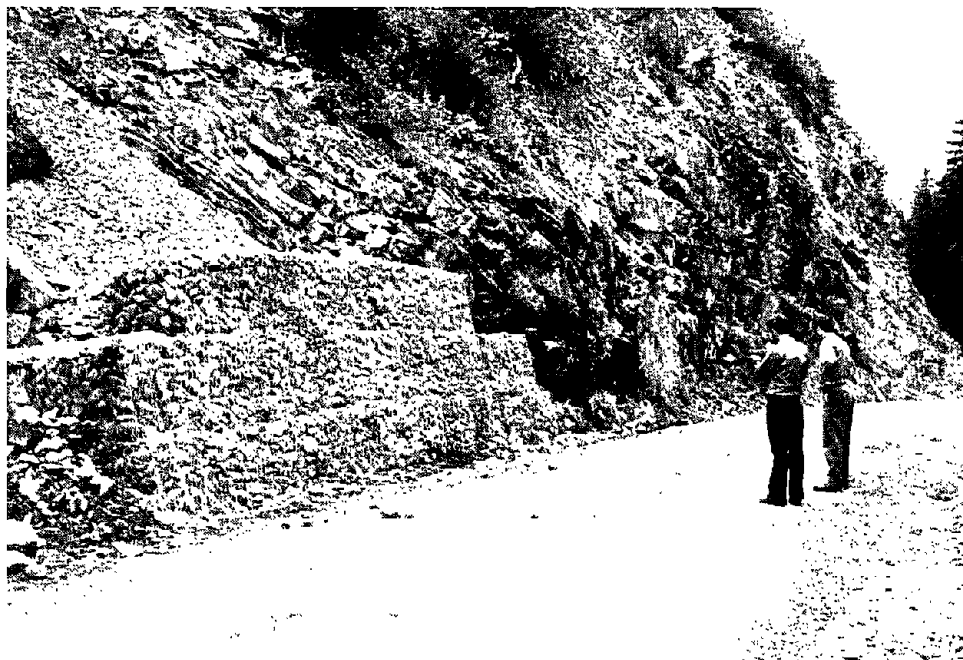
Figure 2-15.—Gabion wall, Quartzville Road Reconstruction, Willamette National Forest.
