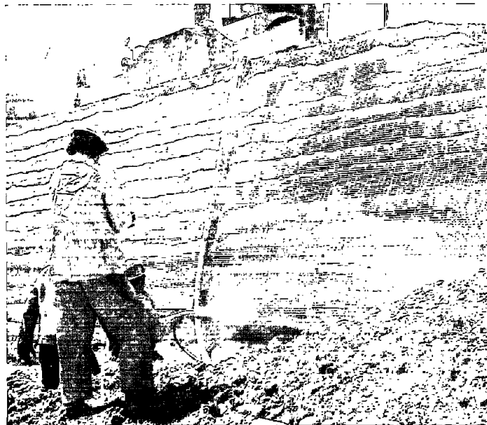
Figure 3.3.—A wrapped-faced wall faced being covered with shotcrete.
